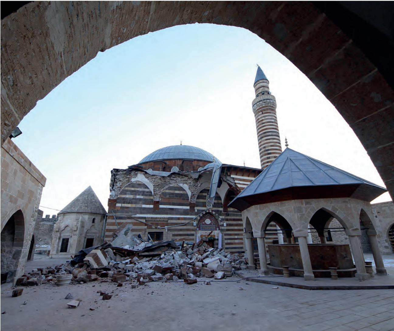
10. The severe damages on the Kaya Çelebi Mosque after the 2011 earthquake in the Upper Bay of Bakracli.
